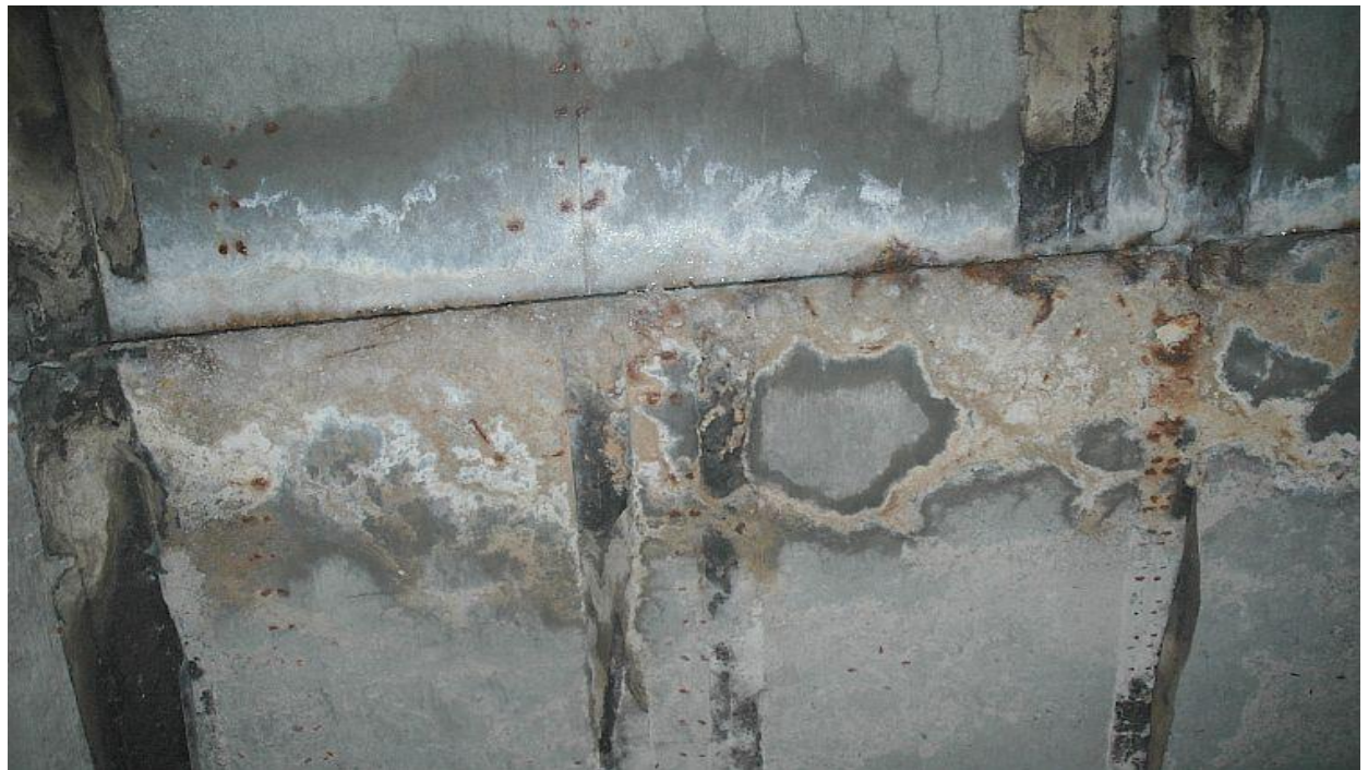
View of Hurricane Creek tunnel ceiling (November 2006)
