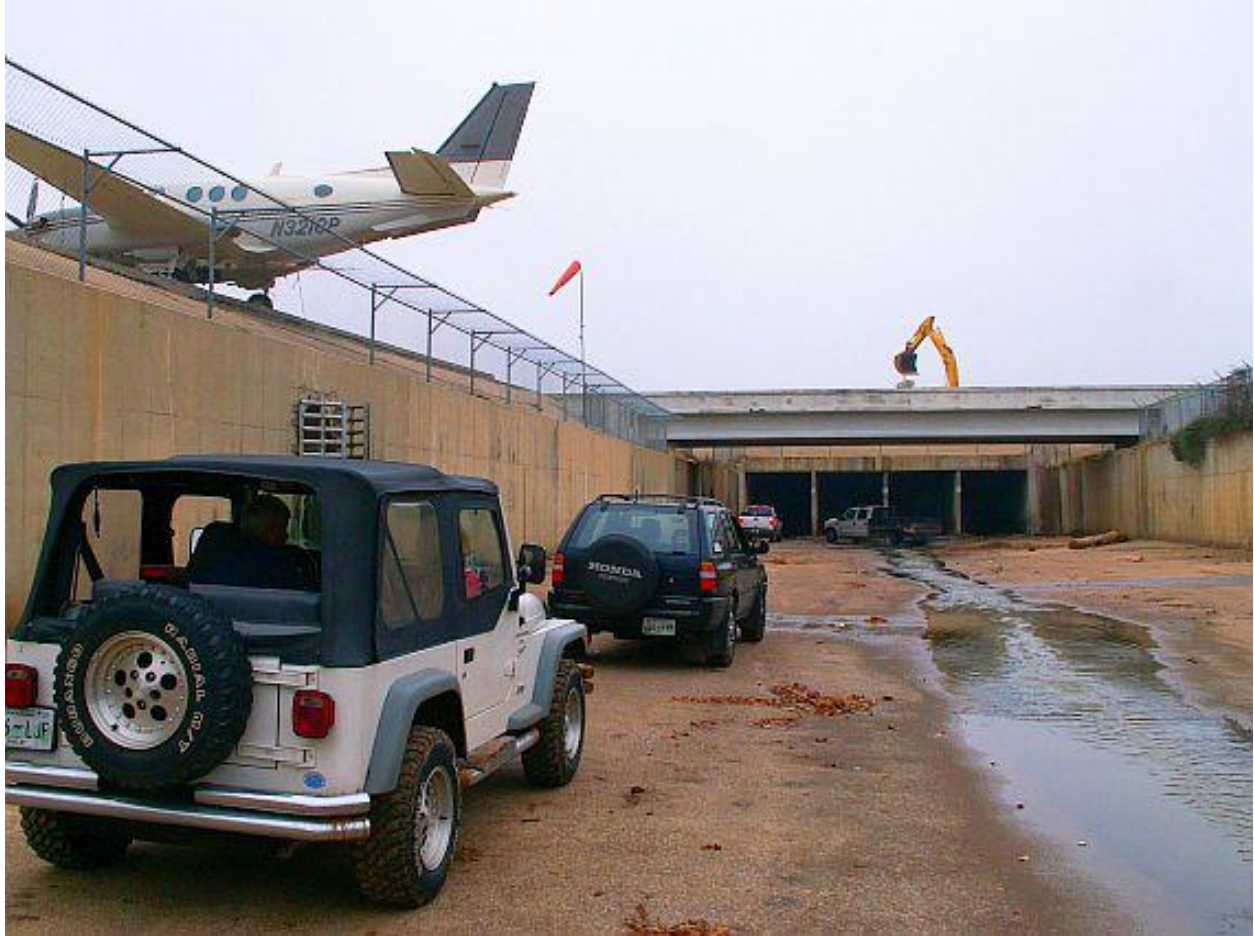
South Entrance to the Hurricane Creek Tunnel
